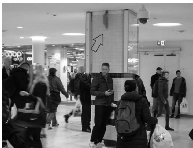
Figure 8. An example of highest exposure area. A man is standing with his smartphone just a couple of meters below a base station (see arrow). In that area maximum measured power density in the GSM +UMTS 900 downlink band was 95,544 \mu\text{W}/\text{m}^2 , which is the upper limit of measurement for EME Spy 200.
